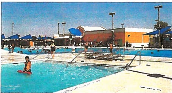
DESIGN & CONSTRUCTION MGMT: CARSON WESTWOOD AQUATIC CENTER - MESA, AZ
