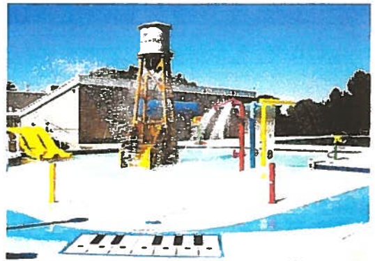
CONSTRUCTION: ANDERSON PARK POOL - WHEAT RIDGE, CO
