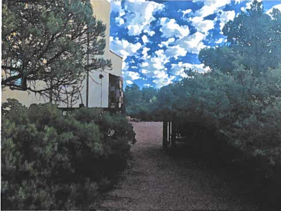
From the South (front) side –
